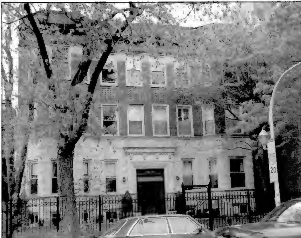
5030-32 North Kenmore Avenue—typical six-flat apartment building (1902)
